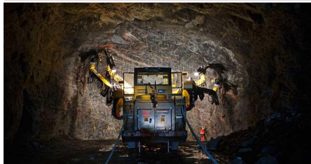
Underground civil engineering
